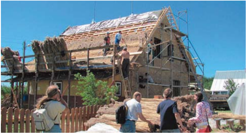
Figure 1. Reed roofing of clay and straw house insulated with reed mats in Zanaroch, June 2010. Photo: E. Shirokov, 2010.
