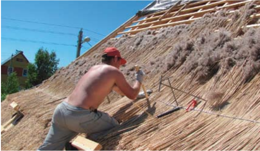
Figure. 3. Reed roofing according to modern technology, Zanaroch, June 2010. Photo: E. Shirokov, 2010.
