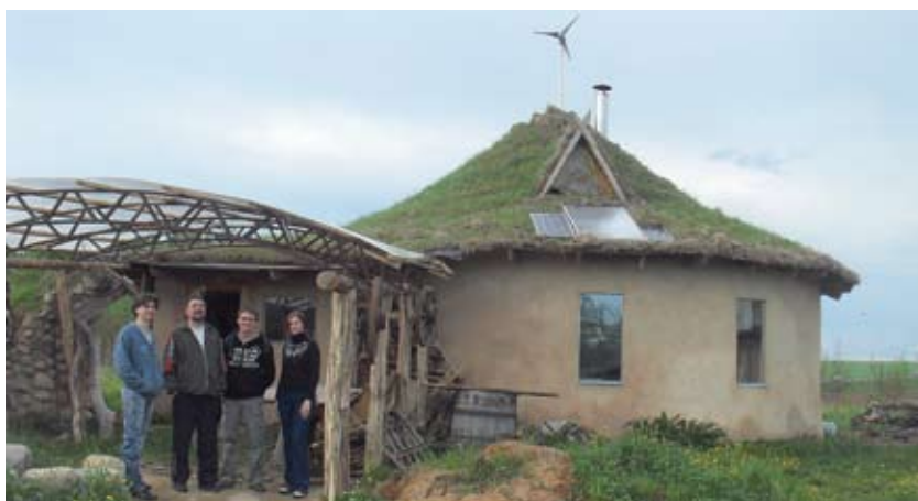
Figure 1. Round 0-Energy straw-bale house in Belaruchi, near Minsk Photo: E.Shirokov, 2010.
