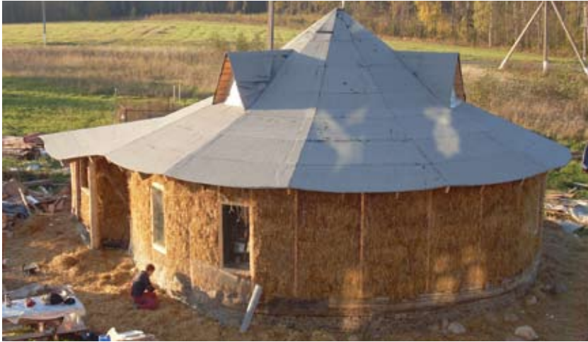
Figure 2. Construction of Round 0-energy straw-bale house Photo: E. Shirokov, 2008.
