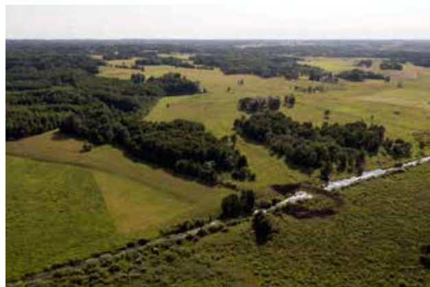
Figure 24. A view of the third dam from above (16.07.2015). Photo: Elm Media
