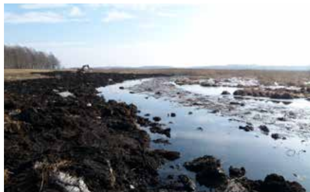
Figure 17. In most sloughy sites at the inflow of the Dviete River into Skuķu lake, the deepening of oxbow was possible only from one bank (20.02.2015). Photo: E. Račinskis
