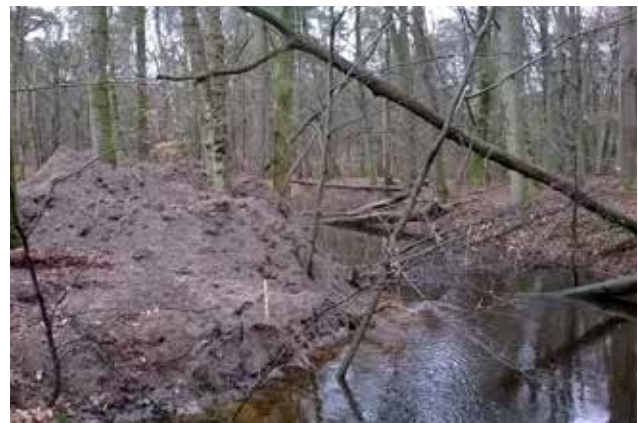
River bed elevation by slowly pushing sand into to the stream, letting the 'water do the work'. Hierdense beek, 2014 (photo: Bart Reeze, Stroming BV).
