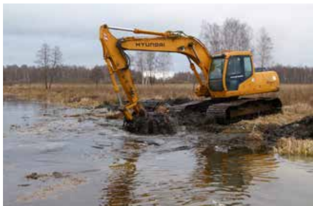
Figure 14. Removal of a beaver dam to decrease the water level for engineering work (14.01.2015). Photo: E. Račinskis
