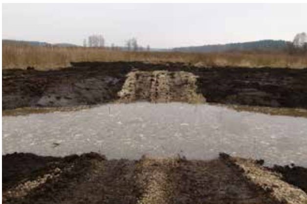
Figure 25. Ford arranged for crossing the river by agricultural machinery (25.03.2015).
