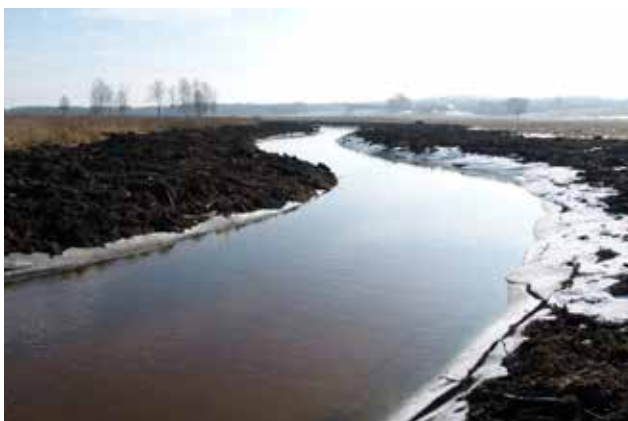
Figure 29. The restored Dviete River soon after excavation (20.02.2015). Photo: E. Račinskis
